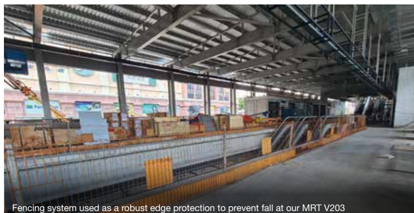
Fencing system used as a robust edge protection to prevent fall at our MRT V203
